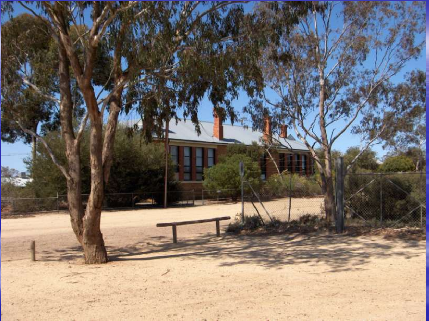
OLD SCHOOL BUILDING
